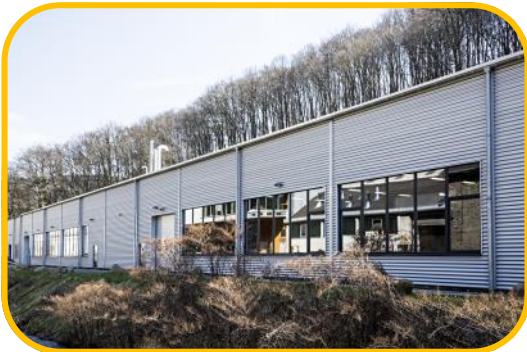
Rhodius Germany Plant
